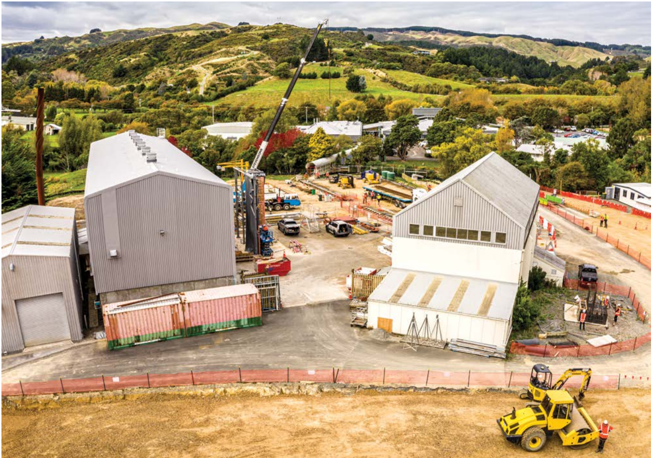
New buildings under construction include state-of-the-art fire and structures laboratories.
